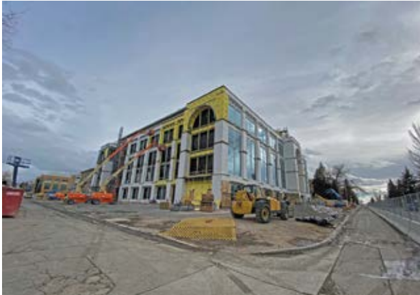
TEAMWORK UW construction and design veterans GE Johnson, GSG Architecture and Perkins+Will teamed up on the $103-million SI building.
