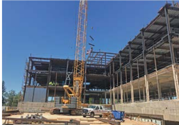
TIME SAVER Concrete cores were placed after the steel framing was erected to shorten the critical path.
